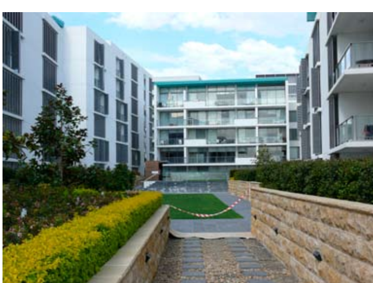
Courtyard apartment housing within internal private spaces
